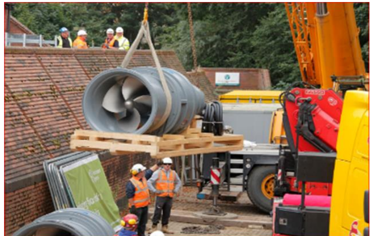
New pump at Foss Barrier
